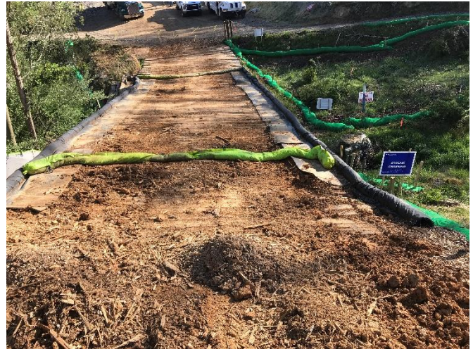
Figure 2: Designated crossing S-NN11, ECD's are in place.
