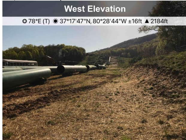
Figure 1: Near St11301+00 pipe is strung and welding crews on site, ECD's are in place.
