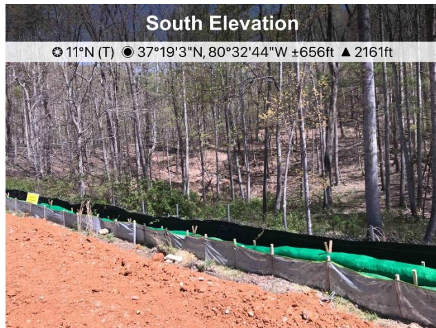
Figure 3: Near St11056 the karsts area is protected by ECD's.
