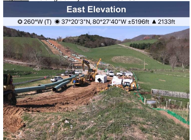
Figure 2: Welding activity near St11493+00.
