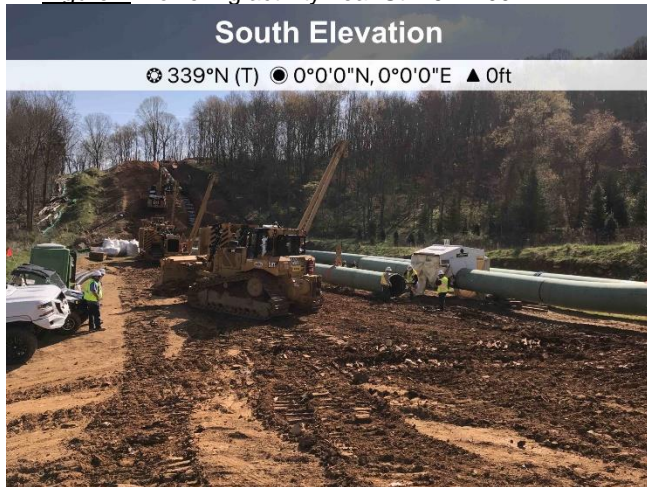
Figure 1: Lowering activity near St11524+00.
