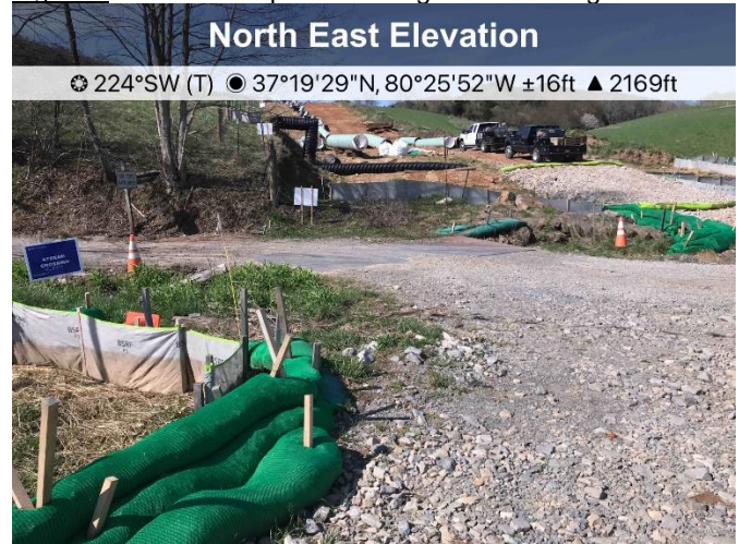
Figure 4: ECD's are in place at designated crossing S-PP1.
