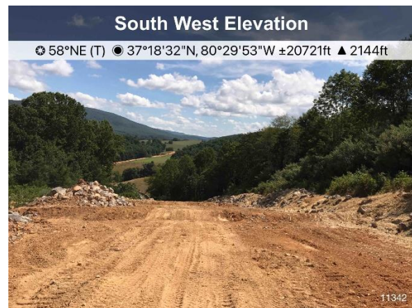
Figure 4: St 11342 ECD's are in place.
