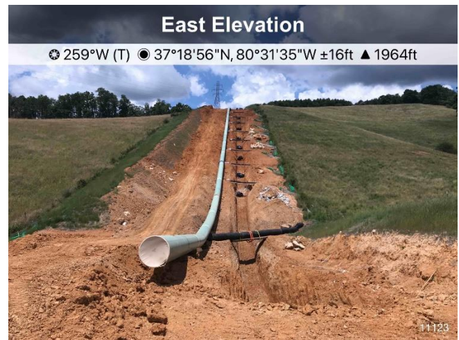
Figure 4: St 11123 ditch has been dug and ECD's are in place
