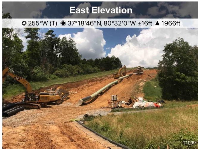
Figure 1: St11099 grading activities, ECD's are in place.
