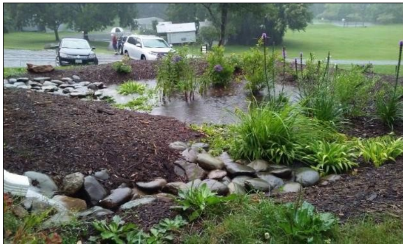
Figure 2: Raingarden BMP (Courtesy of VCAP)
